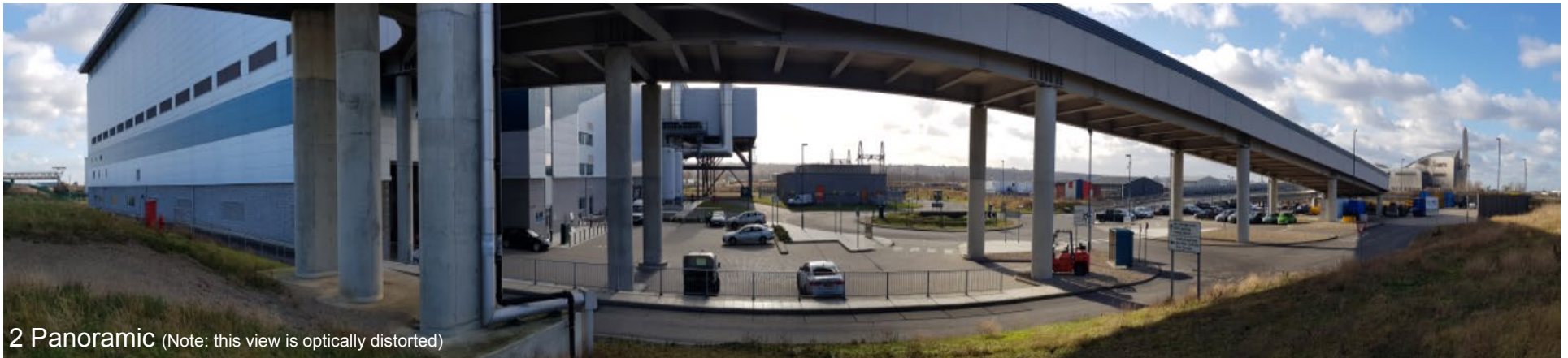
1 Panoramic (Note: this view is optically distorted)
